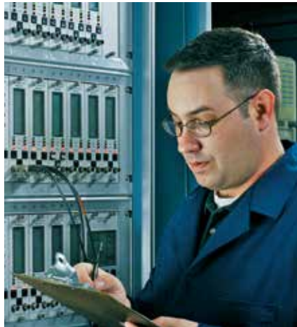
Cameron's test center control room provides computer control of cooling water, input speed and lubricating oil supply.
